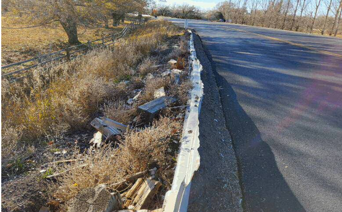
Damaged guardrail with broken posts at SW corner
