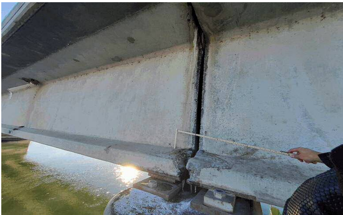
Spalling of girder ends and moisture accumulation from failed seal-girder 1 at pier 1
