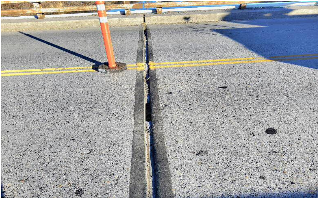
(CS3/CS4) Deteriorated joint over pier (typical)
