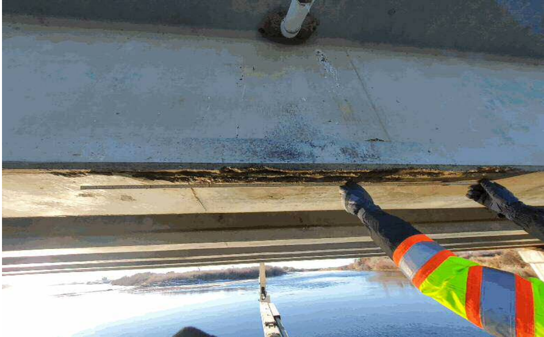
(CS3) Exposed prestress strands at girder 1 bottom-span 2
