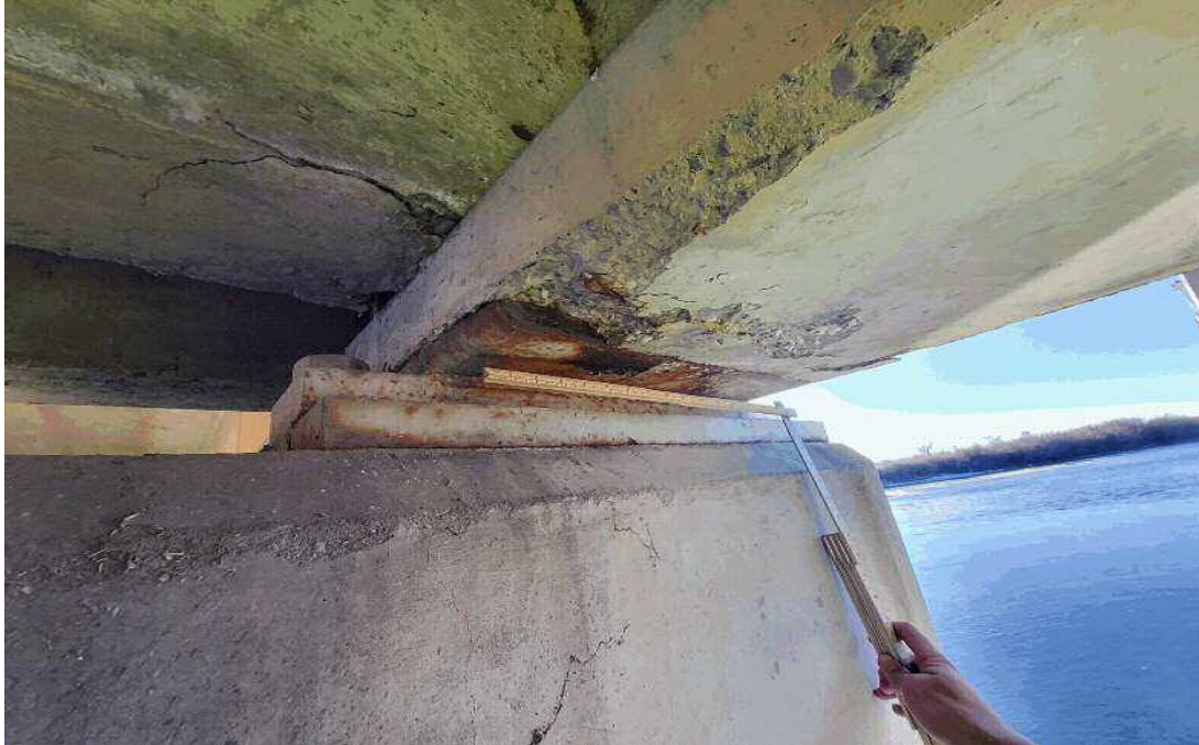
(CS3) Spalling with exposed rebar at girder 5 end-span 1 pier 1
