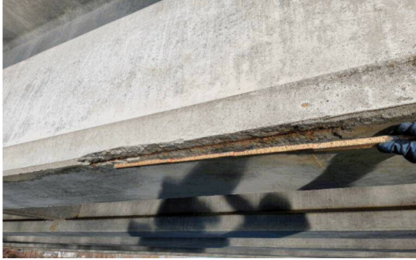
Figure 4: Exposed Prestress Strands at the bottom Girder 5 in Span 2.
