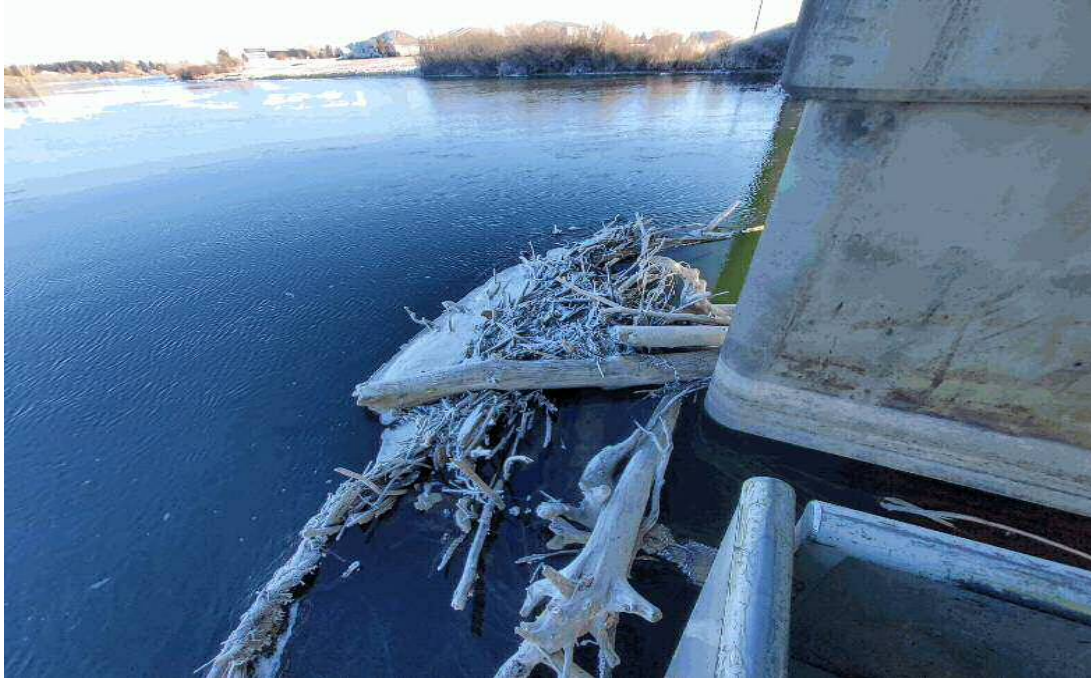
Tree and trapped debris at pier 3 nose
