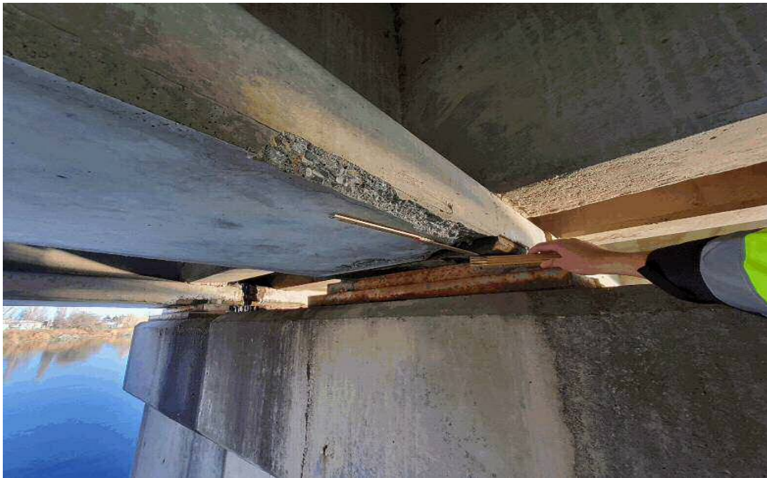
(CS3) Spall at girder 2 end-span 1 pier 1
