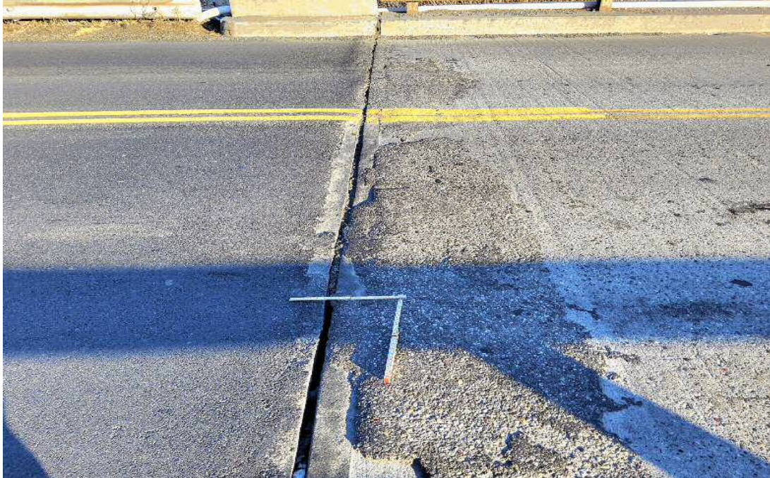
(CS3/CS4) Deteriorated joint at West end
