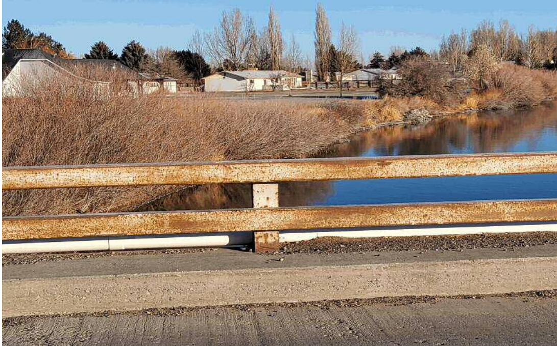
Failed paint on bridge rail
