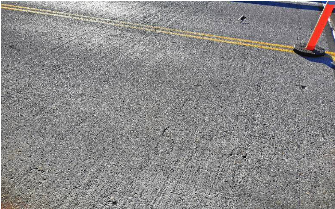
Typical cracking on deck surface
