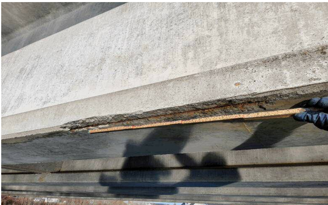
(CS3) Exposed prestress strands at girder 5 bottom-span 2
