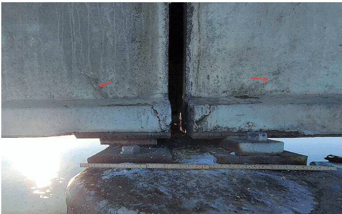
Spalling of girder ends and hairline shear cracking in girder 1 web-pier 2
