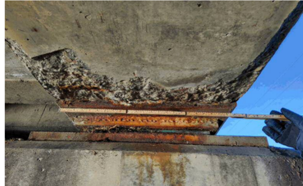
Figure 5: Large Spall with Exposed Rebar at the end of Girder 1, in Span 3. Also Rusting of Bearing at Pier 2.
