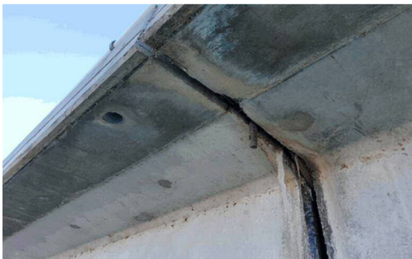
Figure 3: Failed Joint with Leaking Moisture above Pier 1
