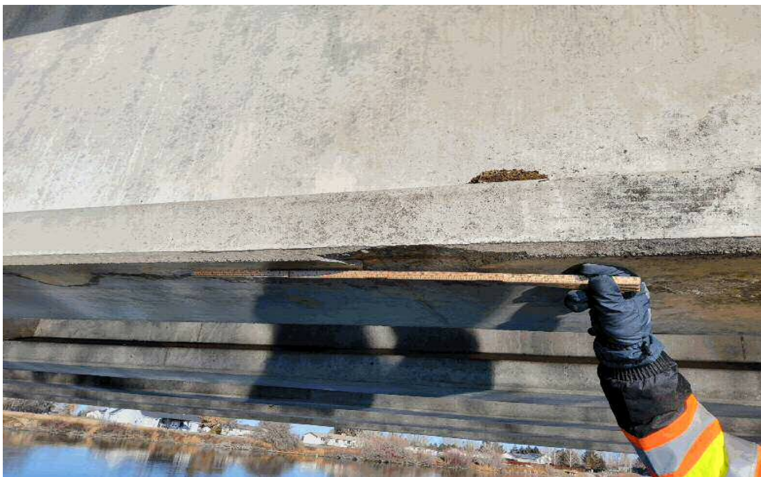
(CS3) Exposed prestress strand at girder 5 bottom-span 4
