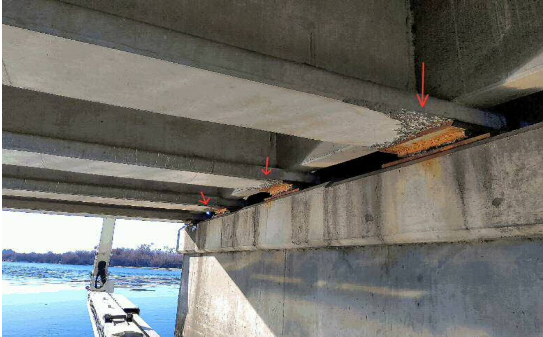
(CS3) Spalling at girder ends-span 5 pier 4
