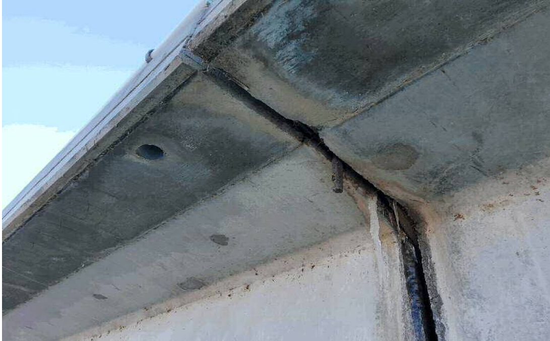
(CS4) Failed joint with leaking moisture above pier 1
