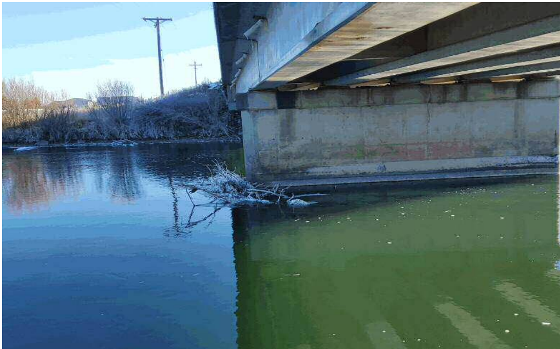
Trapped debris at pier 4 nose
