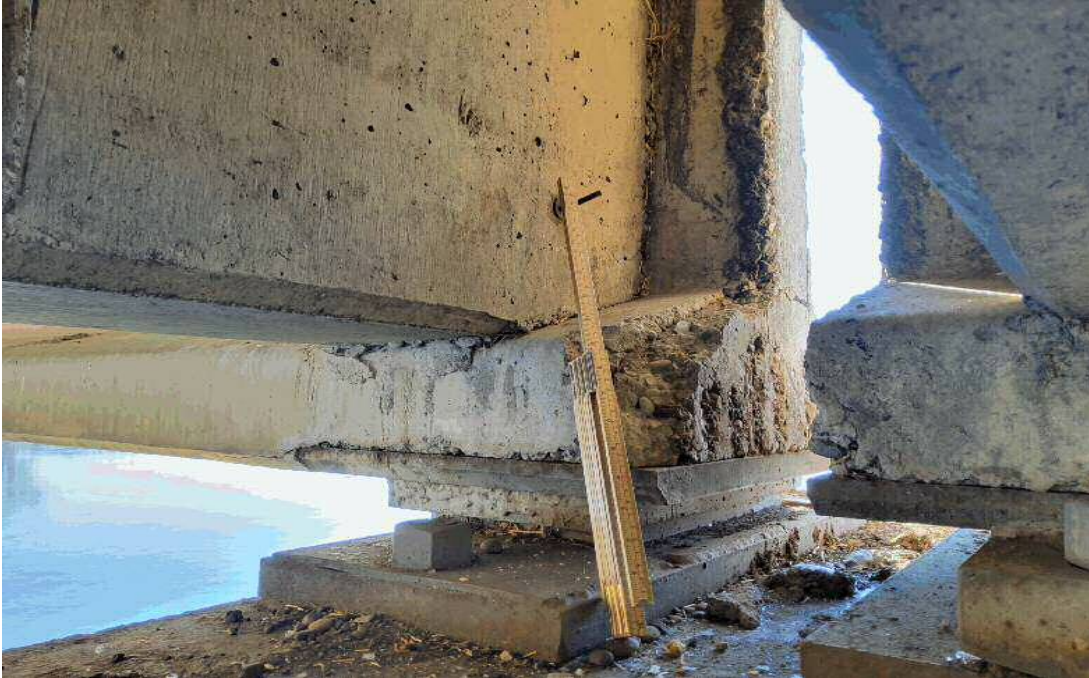
(CS3) Spalling with exposed rebar at girder 5 end-span 3 pier 2
