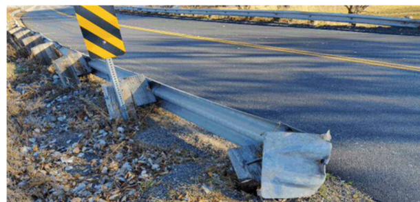
Figure 4: Broken Guardrail from Vehicular Impact at North-west Corner
