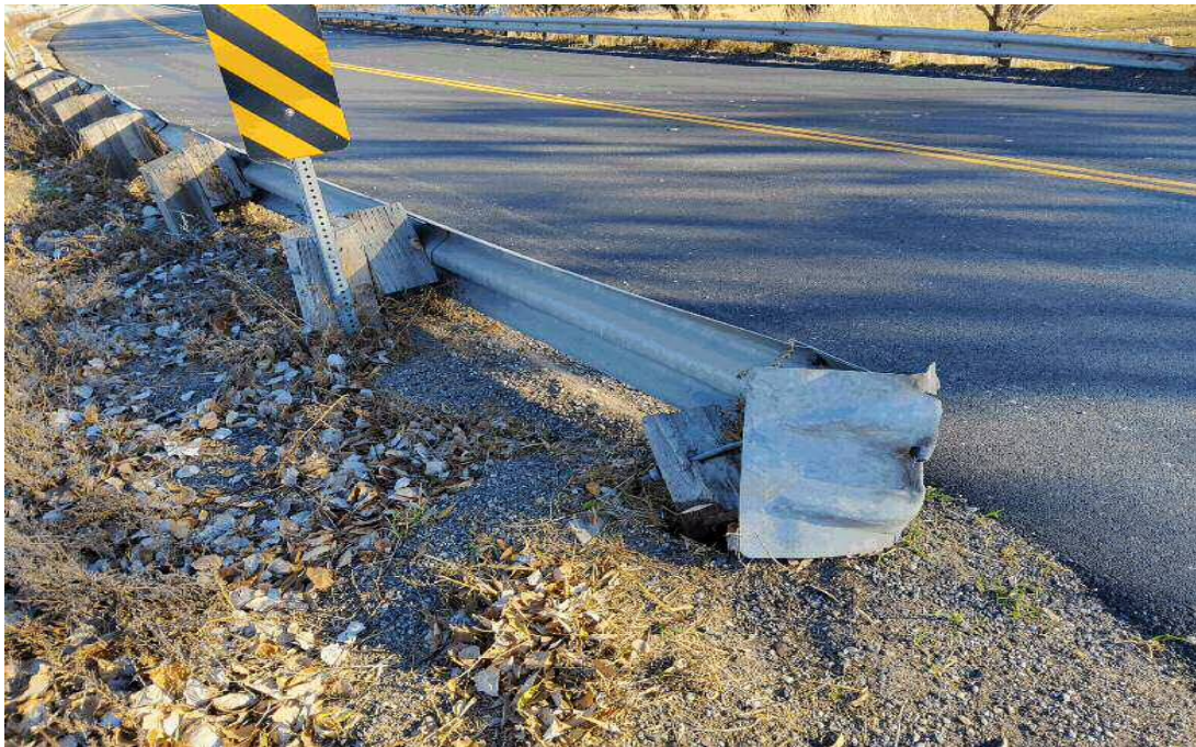
Broken guardrail end post at NW corner
