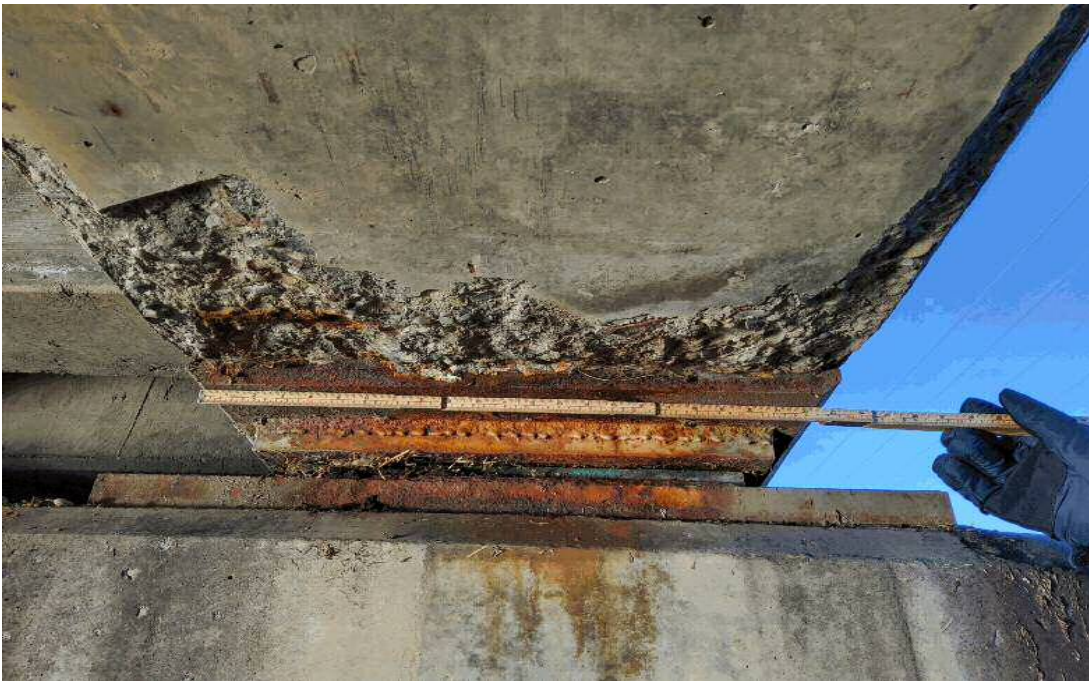
(CS3) Large spall with exposed rebar at girder 1 end-span 3 pier 2-rusting of bearing
